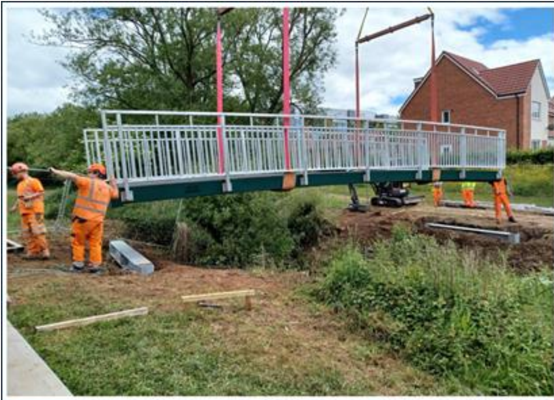
Figure 1-2 - Example Bridge Construction
